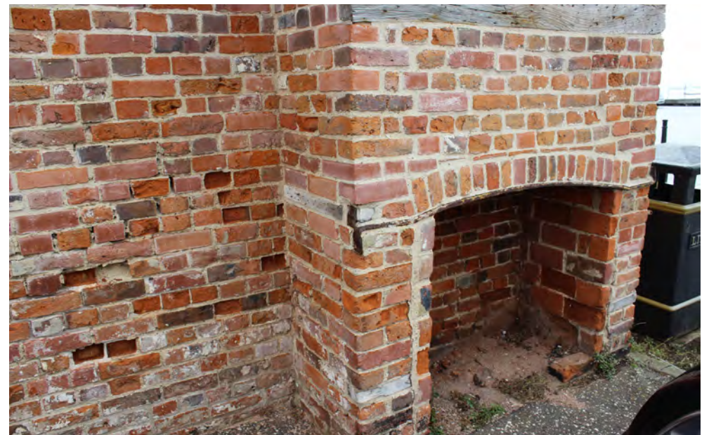
The fireplace in the west external wall of the Custom House
