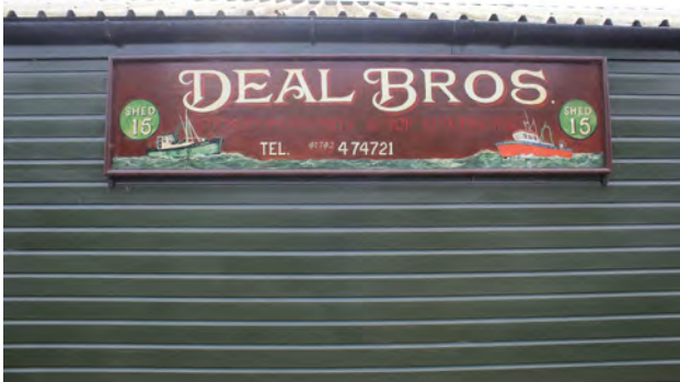
Sensitive signage to one of the cockle sheds
