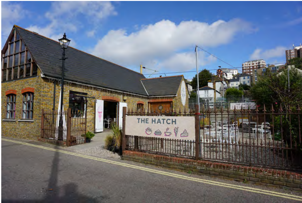
Metal palings outside 66 High Street
